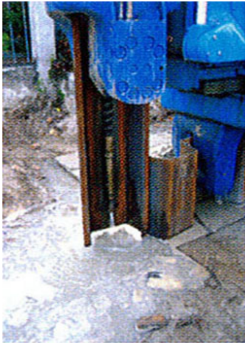
Left: Water jet; Right: Pre-drilling
