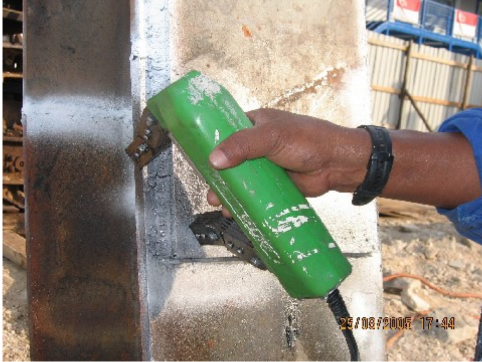
MPI test (Magnetic Particle Inspection) for the welding joint
