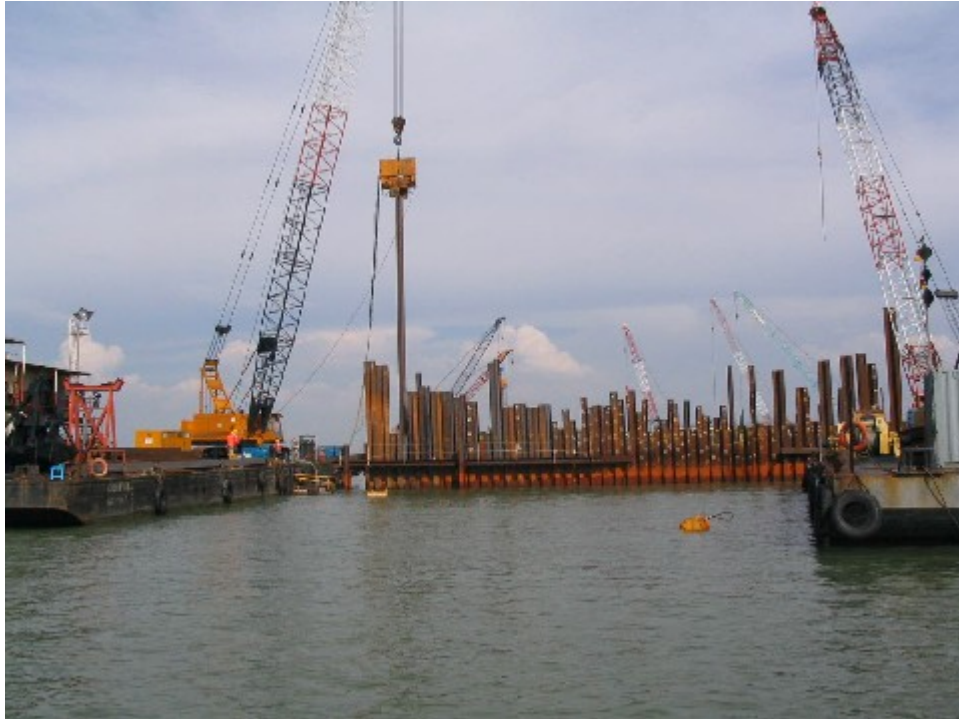
Driving marine sheet pile using vibro hammer from crane barge
