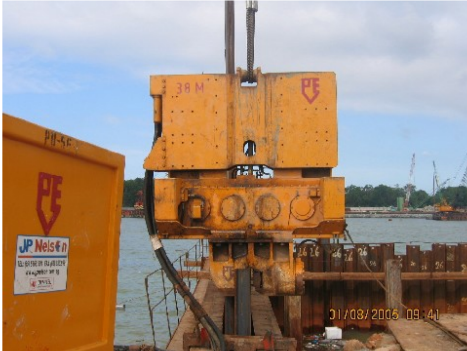
Vibro-driving: A 12-ton vibro hammer
