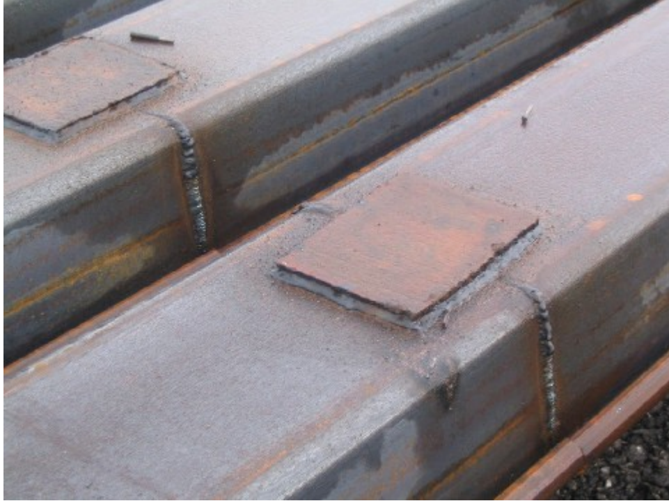
Close view of the sheet pile splicing
