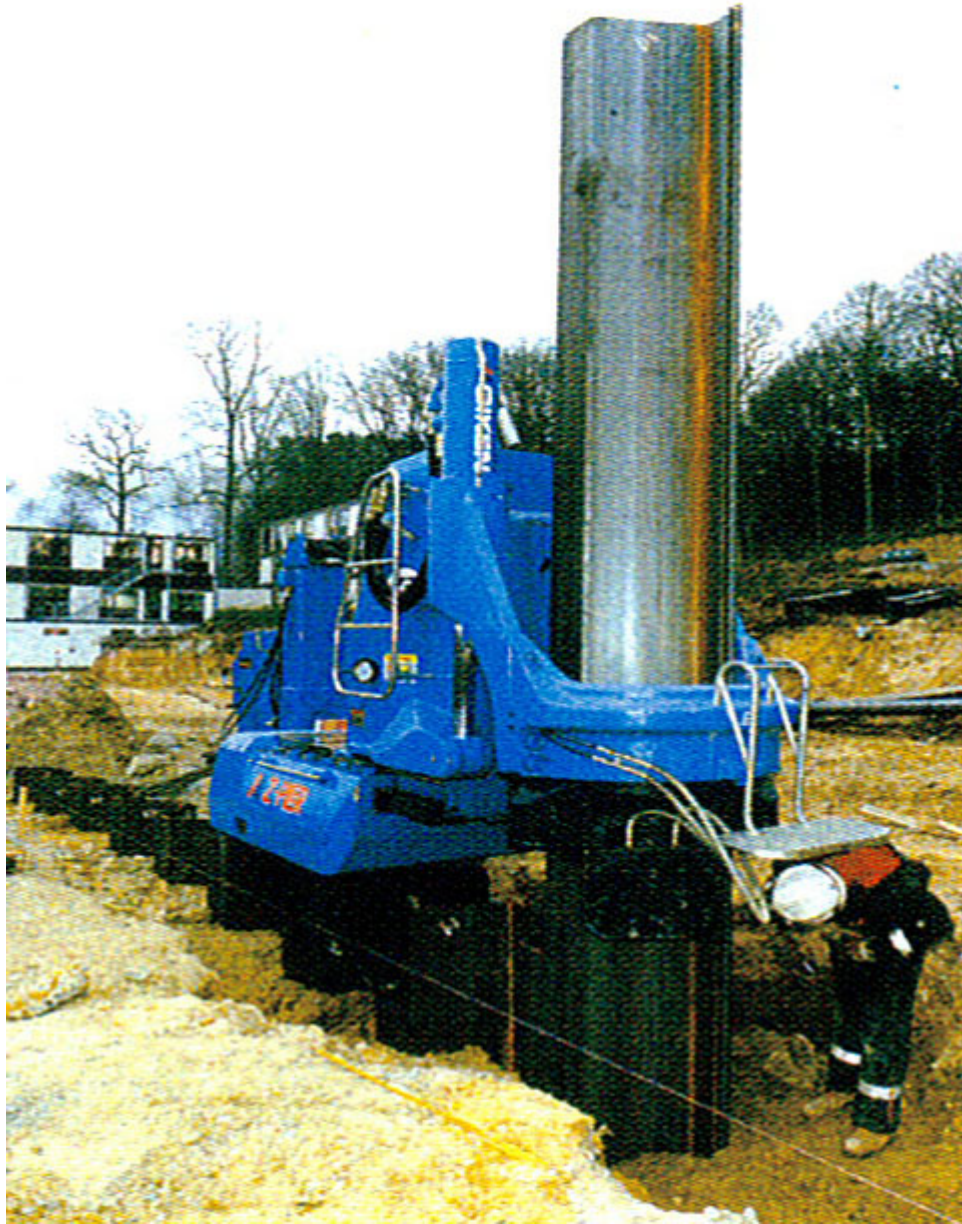
Silent piler for sheet piles
