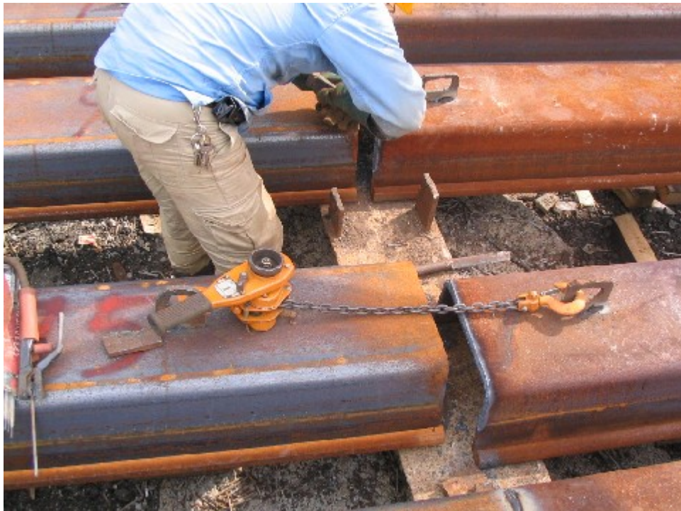
Welding of splicing
