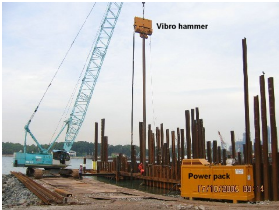
Driving sheet pile using vibro hammer
