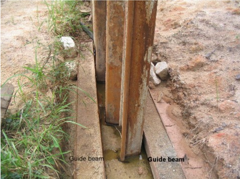
Lay guide beams before installation of sheet piles
